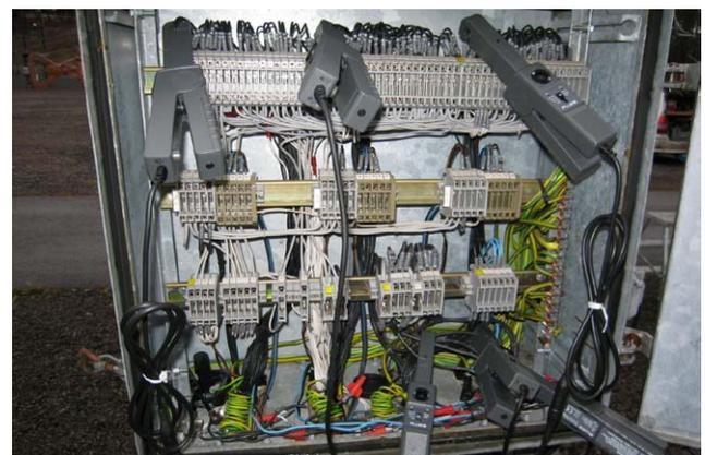
**Figure 3 Control cabinet with current clamps**
