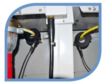
2. PD Cable Monitor<sup>TM</sup> RFCTs simply plug into the UltraTEV Monitor<sup>™</sup>'s multi-sensor nodes.
